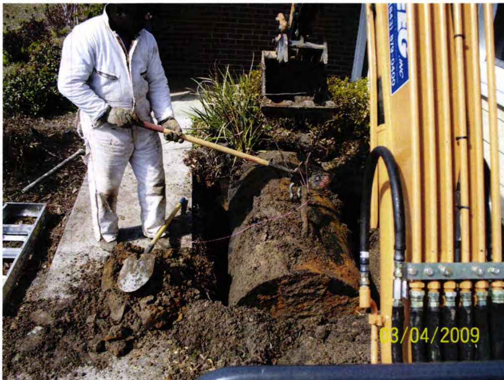
Picture 2: UST 124Banyan-1 during removal.
