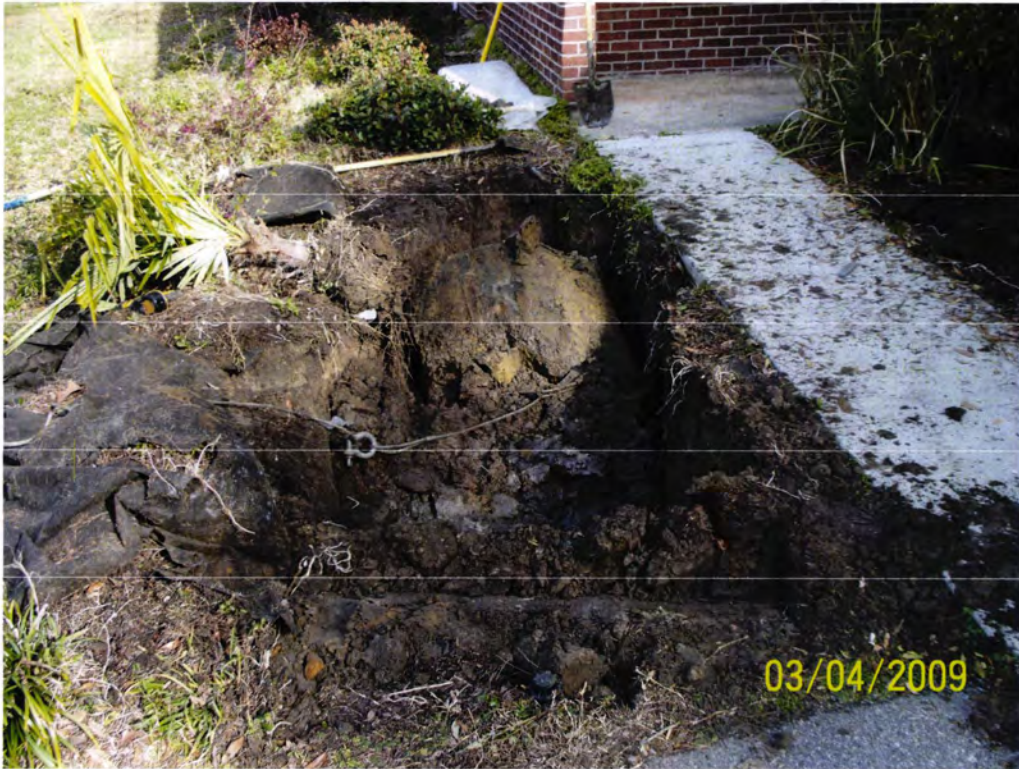
Picture 3: UST 124Banyan-2 during removal.
